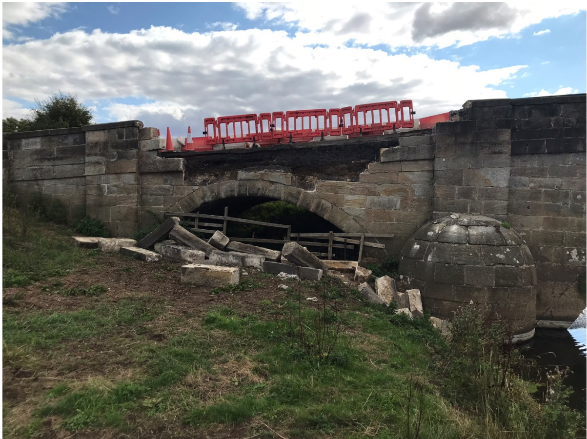
Damage caused to Bubwith bridge after being struck by vehicle on 10 September 2022
